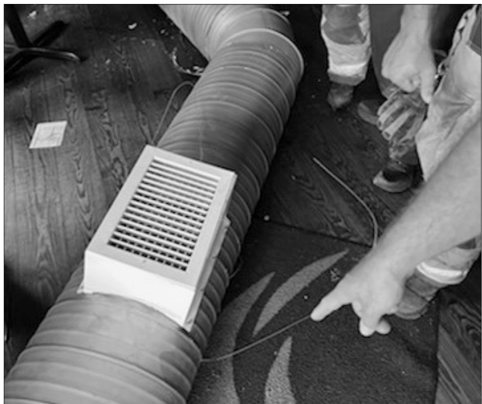
Special | Covington Fire Department It was determined the aircraft cable (pictured), suspending the ductwork from the ceiling inside Mystic Grill, broke and caused the ductwork to fall. No structural damage was found.
