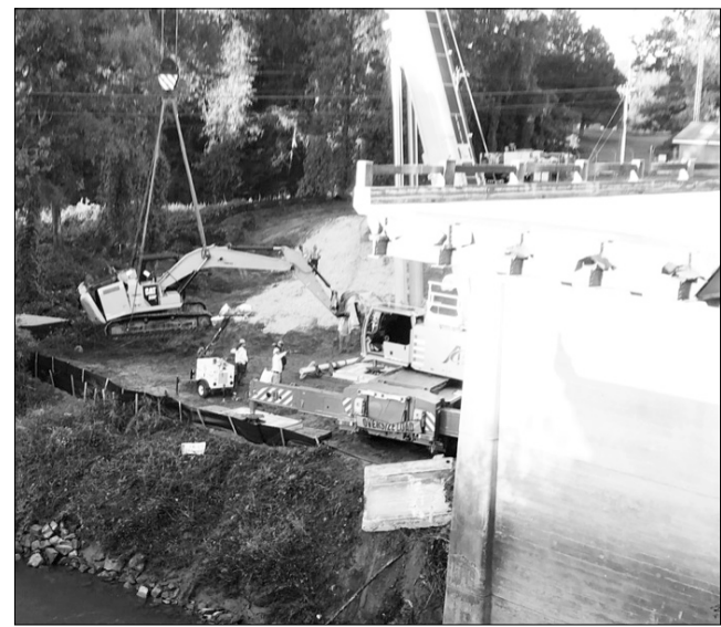
A 500-ton crane is used to lift an excavator from the Yellow River Oct. 20 after the bridge on which the heavy equipment was working collapsed.
